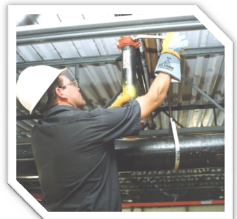
Installing sprinkler pipes
