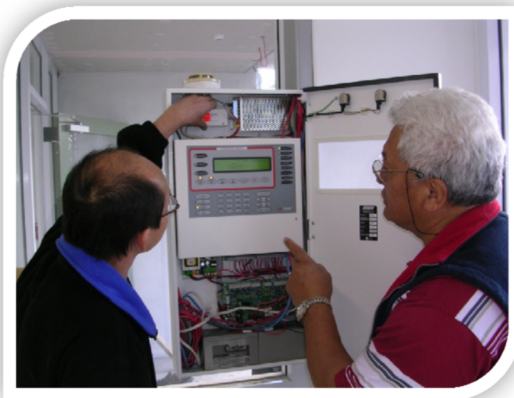
Analogue addressable fire detection and alarm panel
